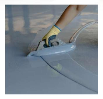
This includes the application of specialized coatings and protective systems to shield structures from environmental, chemical, and mechanical degradation. Common solutions include anti-corrosion coatings for steel reinforcements, epoxy-based coatings for concrete, and protective layers for industrial facilities exposed to aggressive chemicals or high temperatures.
