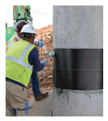
This vertical employs cutting-edge technologies and materials to address a wide array of structural challenges, ensuring cost-effective and efficient solutions. Activities such as crack repair, concrete jacketing, and carbon fiber wrapping not only restore the original strength of structures but often enhance it beyond the initial design capacity. The following scope of treatments highlights the techniques commonly employed:
